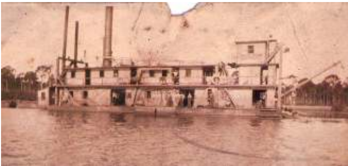
The Clausen Dredge
