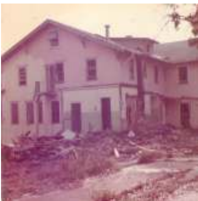
Photos from 1974 demolition
