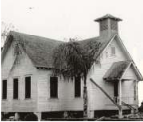
Old Church preparing to move
