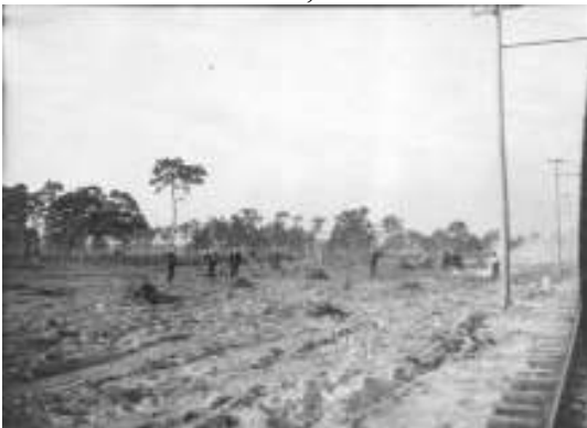
Clearing land next to tracks
