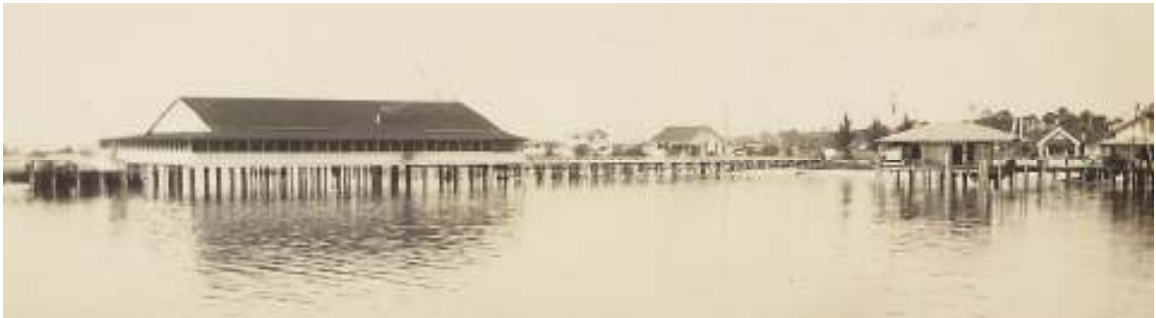
Second Casino, Pier to right
