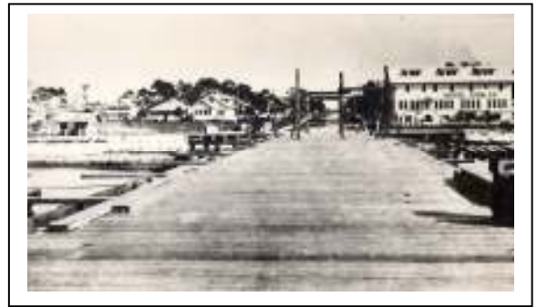
Dobler Hotel at base of pier
