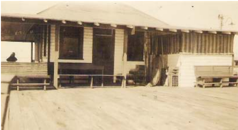
Structure on pier 1920s
