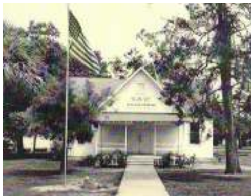
With designation as Archie Tabor Memorial building
