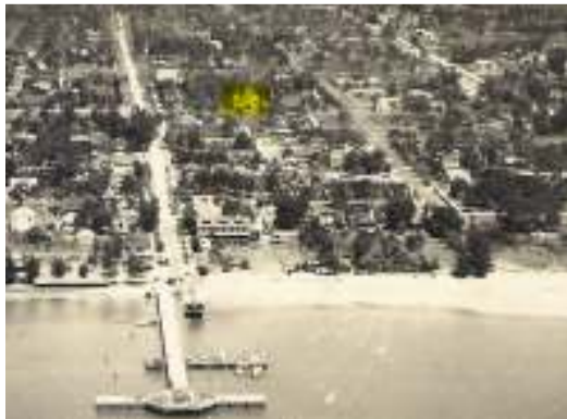
Overview, Showing Location
