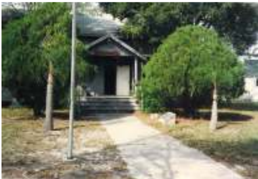
Front Entrance before Restoration
