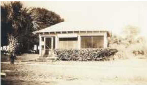
Original library building
